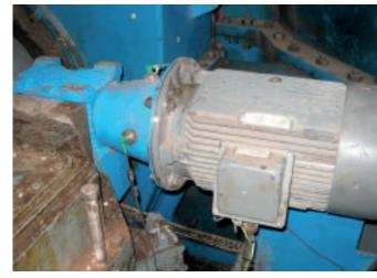
Vibration sensors attached to a steam turbine barring gear box
