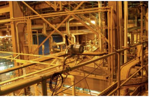
A wireless vibration transmitter mounted outside the turbine enclosure
